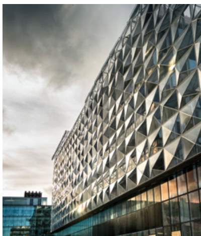
In Denmark, Bravida is installing electrical and heating & plumbing fittings for the Niels Bohr building in Copenhagen
