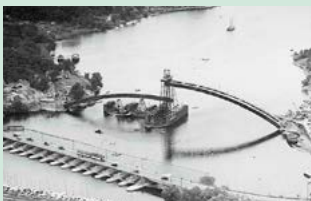
We are involved in the construction of the Traneberg Bridge, work on which starts this year.
